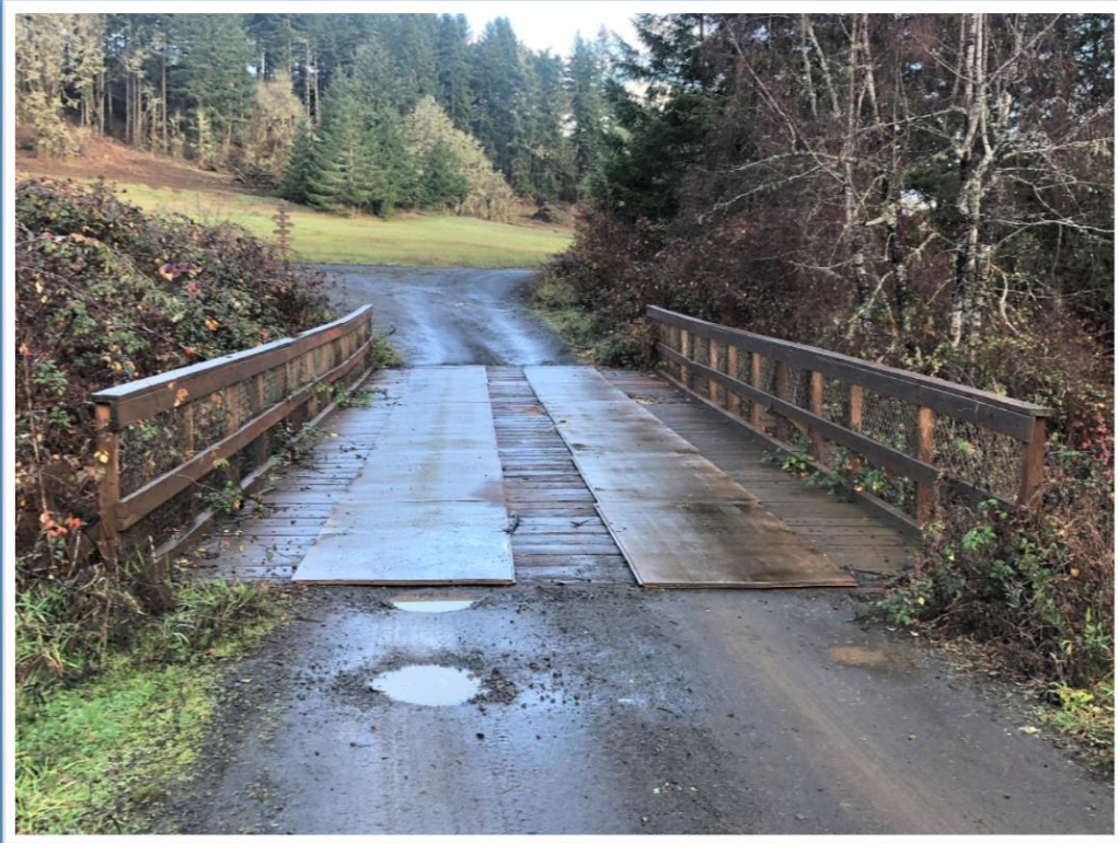
The bridge was weak and compromised
